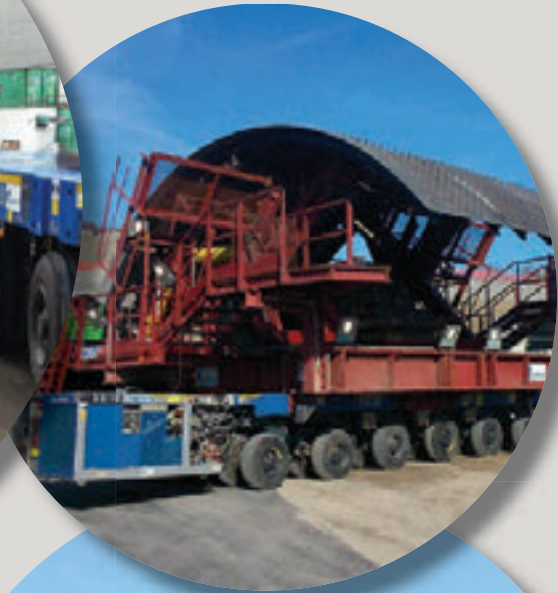
SPARVO TUNNEL REINFORCEMENT A1 HIGHWAY - ITALY
