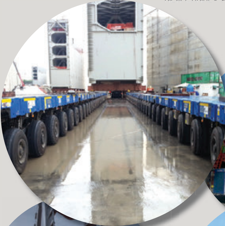
LOCKING GATES NEW CANAL - PANAMA
