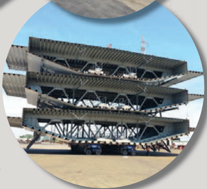
IZMIT BAY CROSSING BRIDGE - TRANSITION SPANS S.GIORGIO DI NOGARO - ITALY
