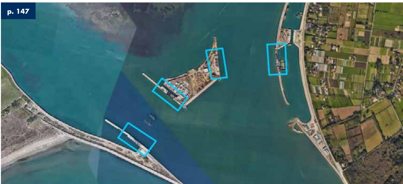
Mose Masking Venice - Italy - 4 independent facilities
