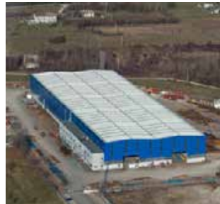
CIMOLAI SpA - Artugna - Italy Total area 87,000 m 2 Covered area 12,000 m 2
