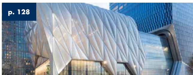
Hudson Yards - The Shed New York - USA - 1,665 m 2 + 1,628 m 2 Covered Area
