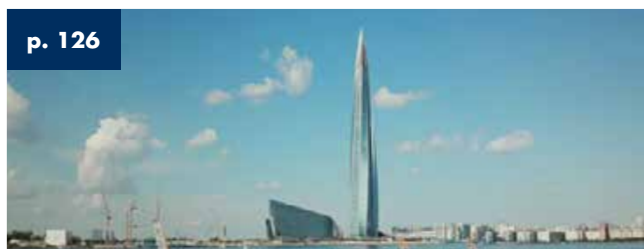
Lakhta Tower St. Petersburg - Russia - 462 m height
