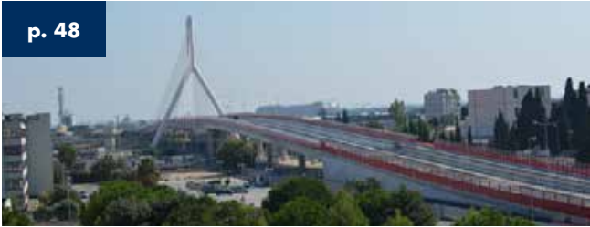
Adriatic bridge Bari - Italy - 626 m total length
