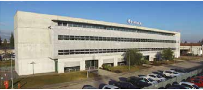
CIMOLAI SpA - Porcia - Italy Administrative offices
