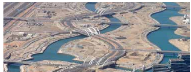
Al Raha bridges Abu Dhabi - UAE - 80 m - 88 m total length 2011
