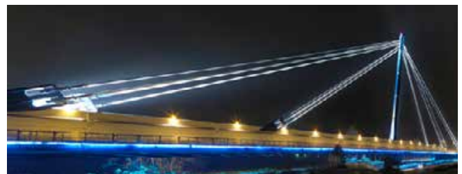
Cable Stayed bridge over the Adda river Montodine - Italy - 400 m total length 2003
