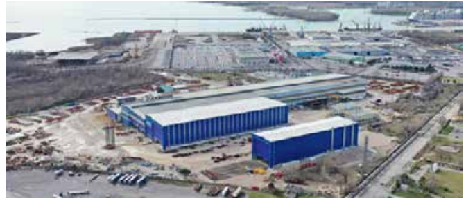
CIMOLAI SpA - Monfalcone - Italy Total area 280,000 m 2 - 60,000 m 2 covered area
