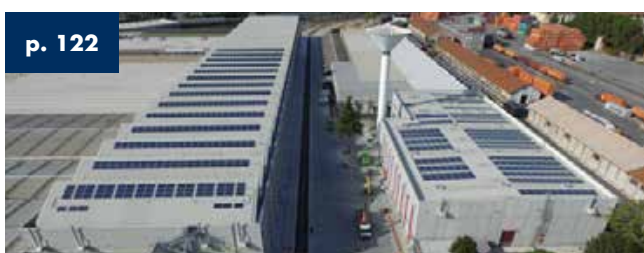
Reconstruction of the OMC factory Vicenza - Italy - 140,000 m 2 covered area
