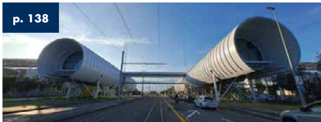
p. 138 Cern New Gateway Geneva - Switzerland - 2.060 m 2 glass facades 2023
