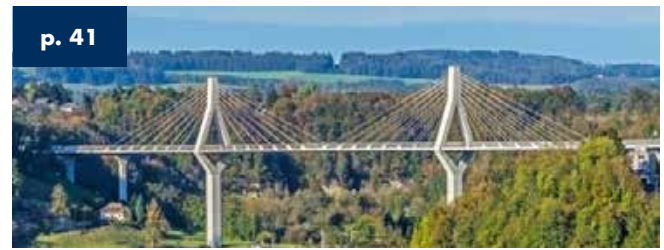
Poya viaduct Fribourg - Switzerland - 850 m total length 2013
