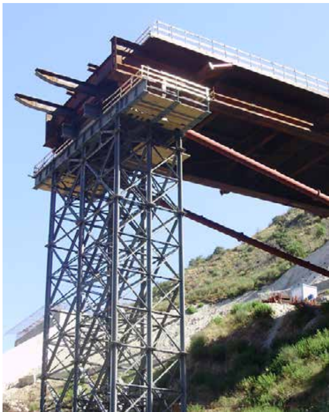
TEMPORARY TOWERS - with cross or circular sections
