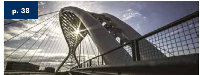
Ostiense bridge Rome - Italy - 160 m total length 2011
