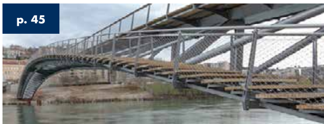
Footbridge over the Rhone Lyon - France - 260 m total length 2013
