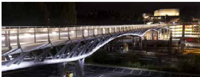
Viaduct Leon Blum Poitiers - France - 310 m total length 2013
