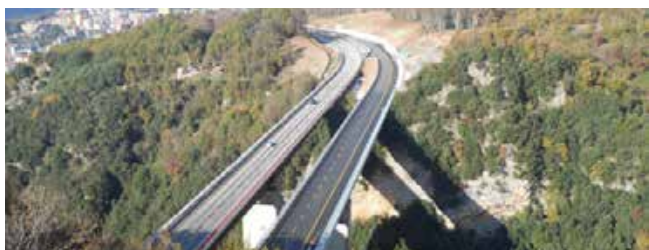
Serra viaduct A3 motorway - Italy - 230 m total length 2014
