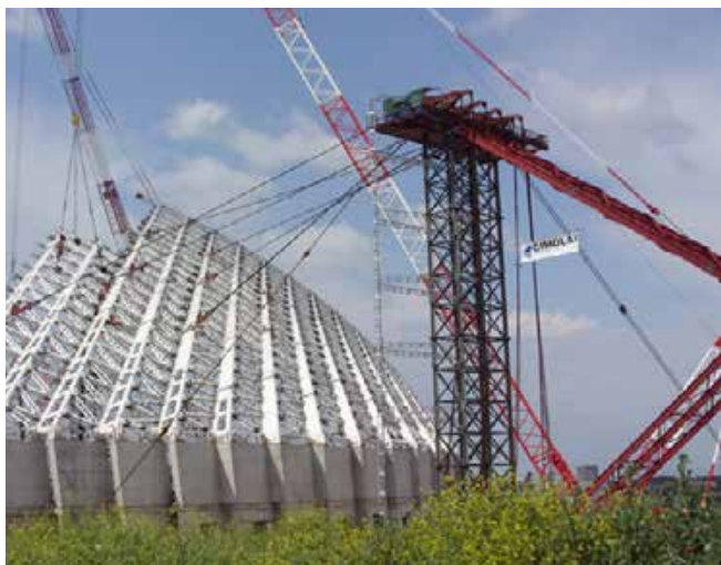
TEMPORARY TOWERS - with cross or circular sections
