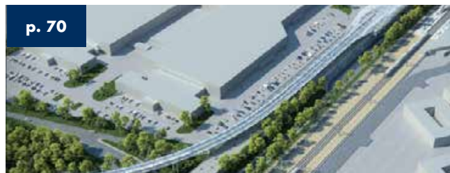
Line 17 Paris Metro 2023 Paris - France - 3,4 km of viaduct
