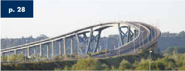
Viaduct over the Grand Canal Maritime Le Havre - France - 1,410 m total length 1994
