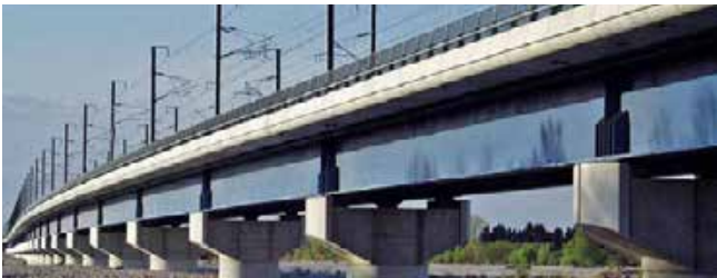
Cavillon Viaduct e Cheval Blanc Cavillon - France - 2,500 m total length 1997
