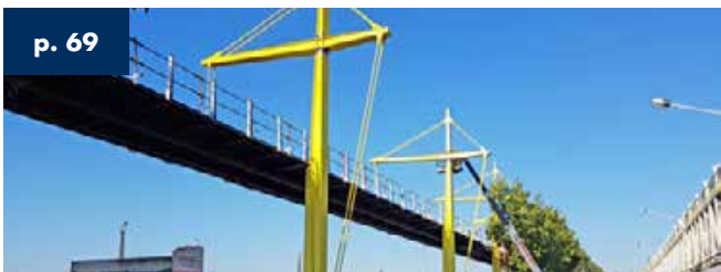
Cyclist Footbridge PC8 2023 Esch Sur Alzette - Grand Duchy of Luxembourg - 1,700 m total length
