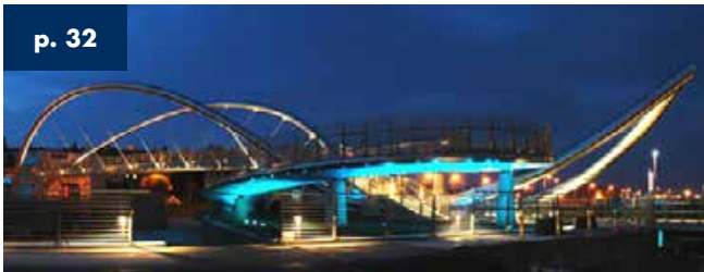
p. 32 Celtic Gateway bridge Holyhead - UK - 170 m total length 2006
