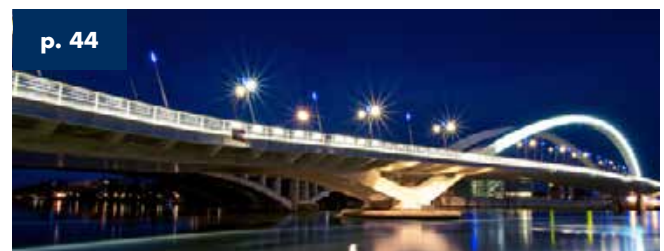
Raymond Barre bridge Lyon - France - 260 m total length 2013
