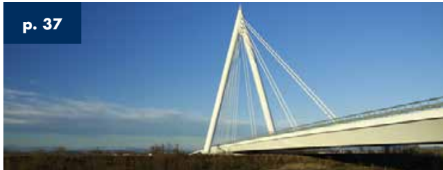
Viaduct over the Adige river South Val d'Astico - Italy - 1,000 m total length 2010
