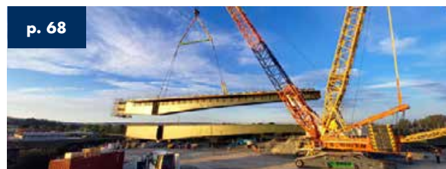
N69 River Feale Bridge 2023 Kerry - Republic of Ireland - 7 km of road
