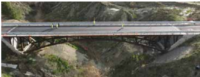
Pisticci bridge Matera - Italy - 60 m total length
