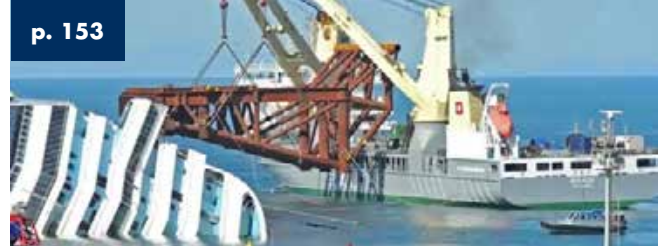
Costa Concordia removal platforms Giglio island - Italy - 35 m x 45 m x 20 m dimension
