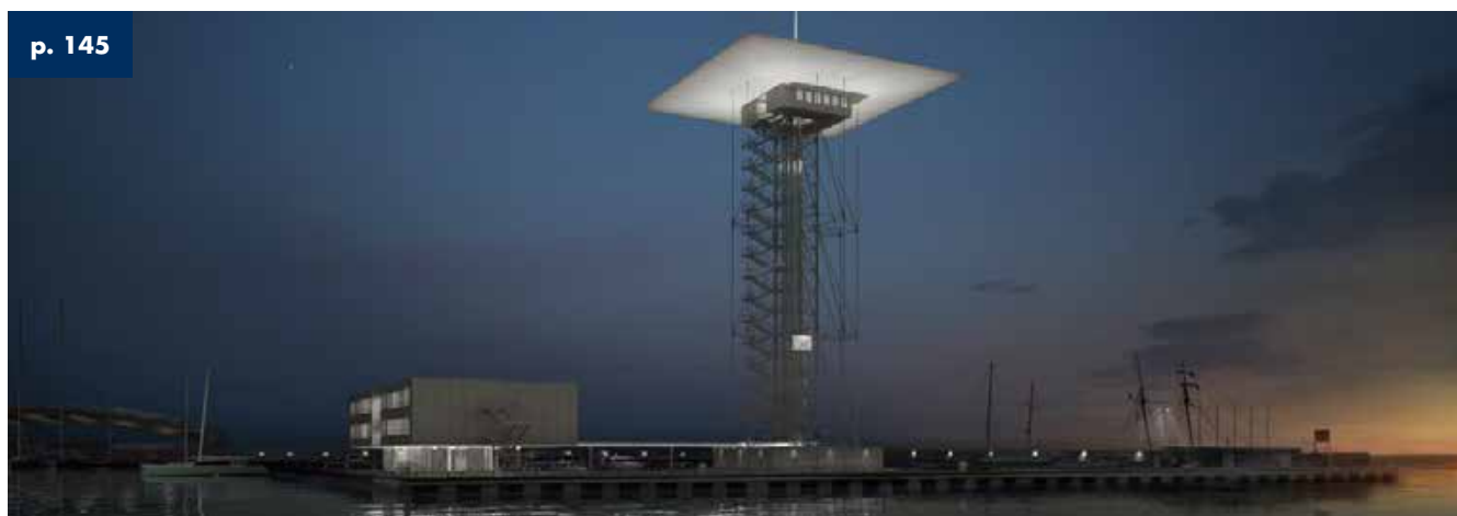
Pilots Tower Genova - Italy - 65 m height
