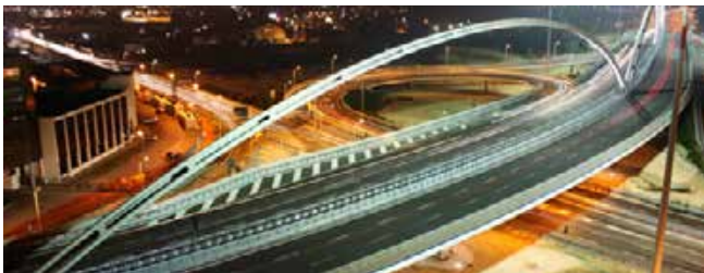
Darwin bridge Padova - Italy - 550 m total length 2008
