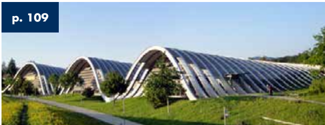
p. 109 Paul Klee center Bern - Switzerland - 12,000 m 2 covered area 2003
