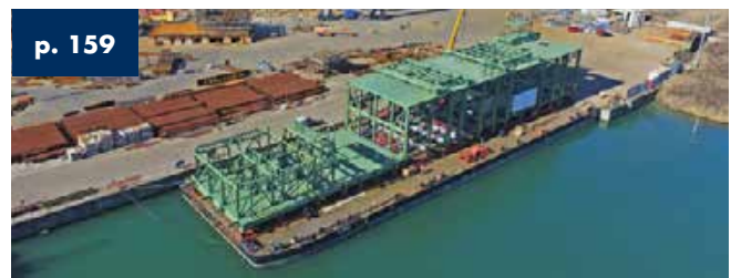
On Shore structures - Tengiz Kazakhstan - 20 modules
