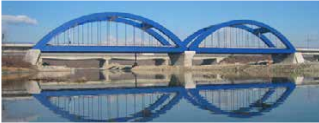
Railway bridge over Dora Baltea Rondissone - Italy - 150 m total length 2004
