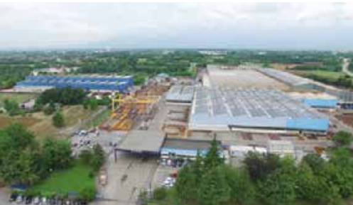
CIMOLAI SpA - Roveredo in Piano - Italy Total area 121,000 m 2 - Covered area 50,500 m 2
