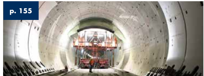
Sparvo tunnel A1 motorway - Italy - 540 m total length
