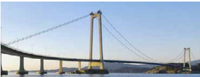
Bomla bridge Stord - Norway - 500 m total length 2000
