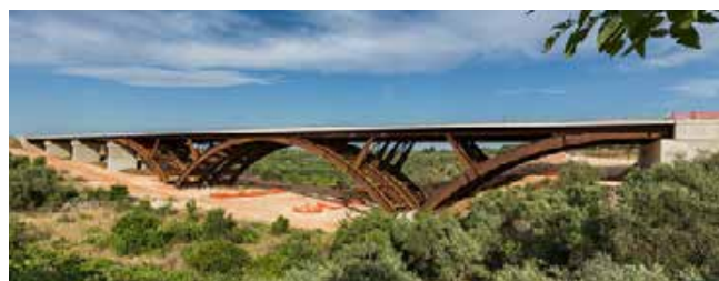
Lame Strette bridges Bari - Italy - 1,205 m total length 2016
