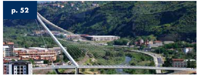
Bridge over the Crati river Cosenza - Italy - 140 m total length
