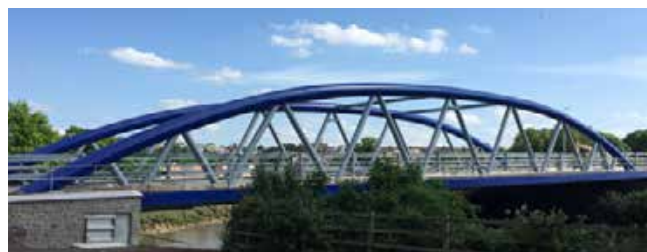
Temple Quay bridge Bristol - UK - 65 m total length 2016
