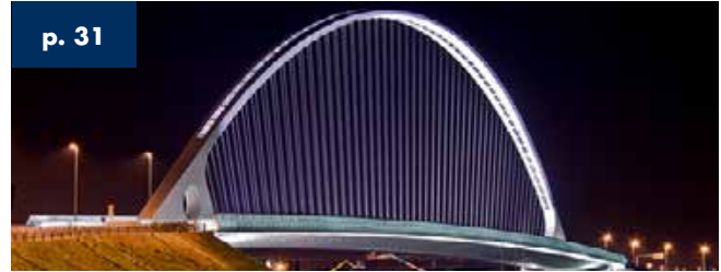
p. 31 Viaducts in Reggio Emilia A1 motorway - Italy - 220 m - 180 m total length 2006
