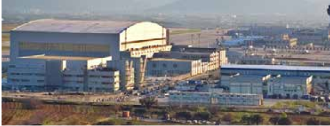
Airport maintenance hangar Athens - Greece - 24,000 m 2 covered area 2001
