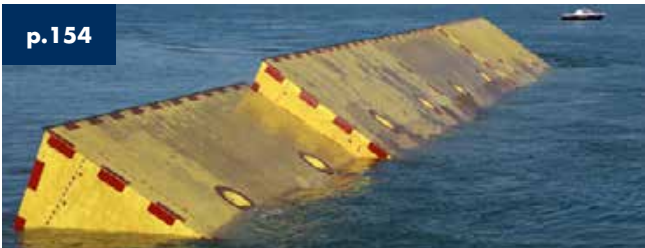
Mo.s.e. - Lido Port Entrance Venice - Italy - 23 gates
