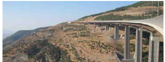
Viaducts on the Adana-Gaziantep motorway Turkey - 5,200 m total length 1999
