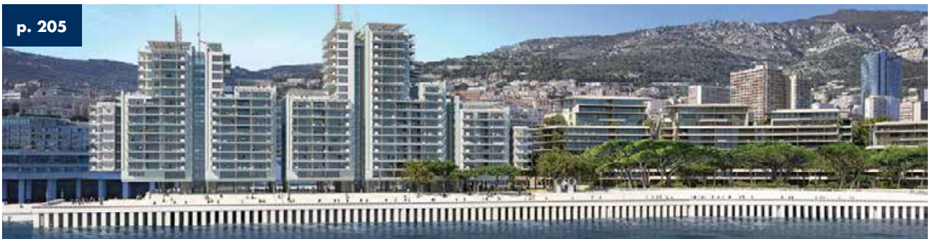
Mareterra Monaco - Principality of Monaco - aluminum cladding - 17,000 m 2
