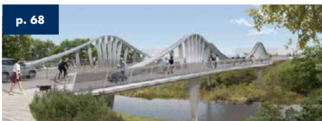
16 Tech Bridge 2023 Indianapolis - USA - 207 m total length
