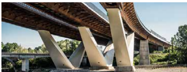
Viaducts over the Lambro river A1 motorway - Italy - 4,000 m total length 2016
