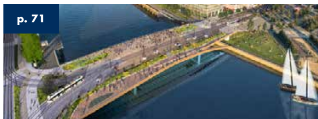
Anne De Bretagne Bridge 2023 Gonesse - France - 140 m total length
