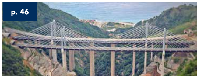
Favazzina viaducts A3 motorway - Italy - 440 m total length 2013
