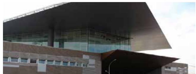
Tiburtina railway station Rome - Italy - 50,000 m 2 covered area 2011
