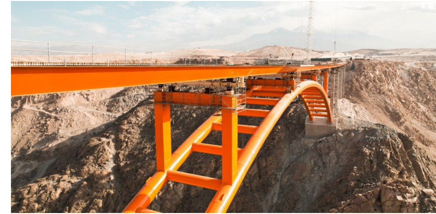
La Joya Bridge & Viaduct 2022 Arequipa - Peru
