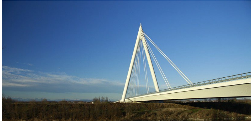
Viaduct over Adige river 2010 Sud Valdastico - Italy
