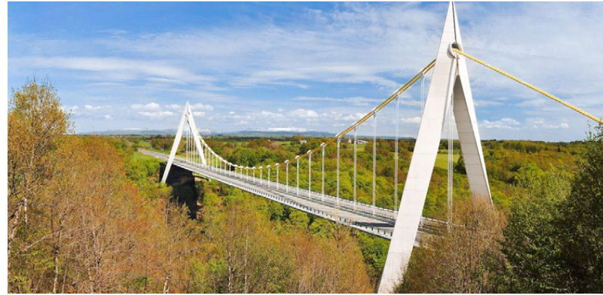
Chavanon Viaduct 2001 Merlines - France
