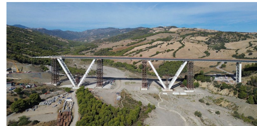
S.S. 106 Jonica Ongoing Calabria - Italy
