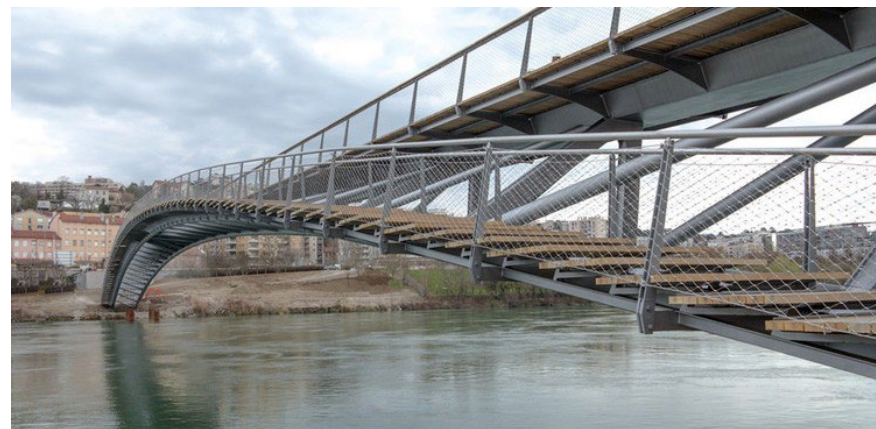
Pedestrian Bridge over the Rhone 2013 Lyon - France
