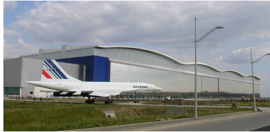
Airbus Assembly Hangar 2003 Toulouse - France
